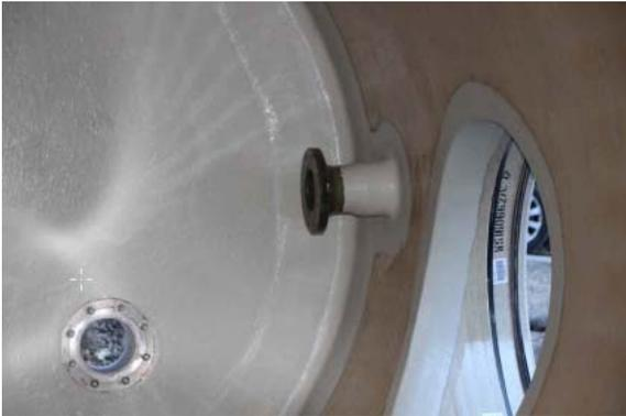
The necessary entries, flanges, sleeves or pipe connections can already be fitted to the elements in the factory.
