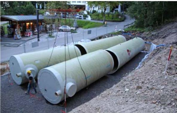
The 6 m long pipe sections complete the FLOWTITE GRP water storage system totalling 18 m in length with a total capacity of 160 m<sup>3</sup>.
